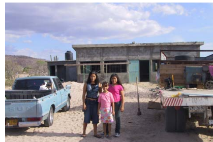
The dining room being constructed
